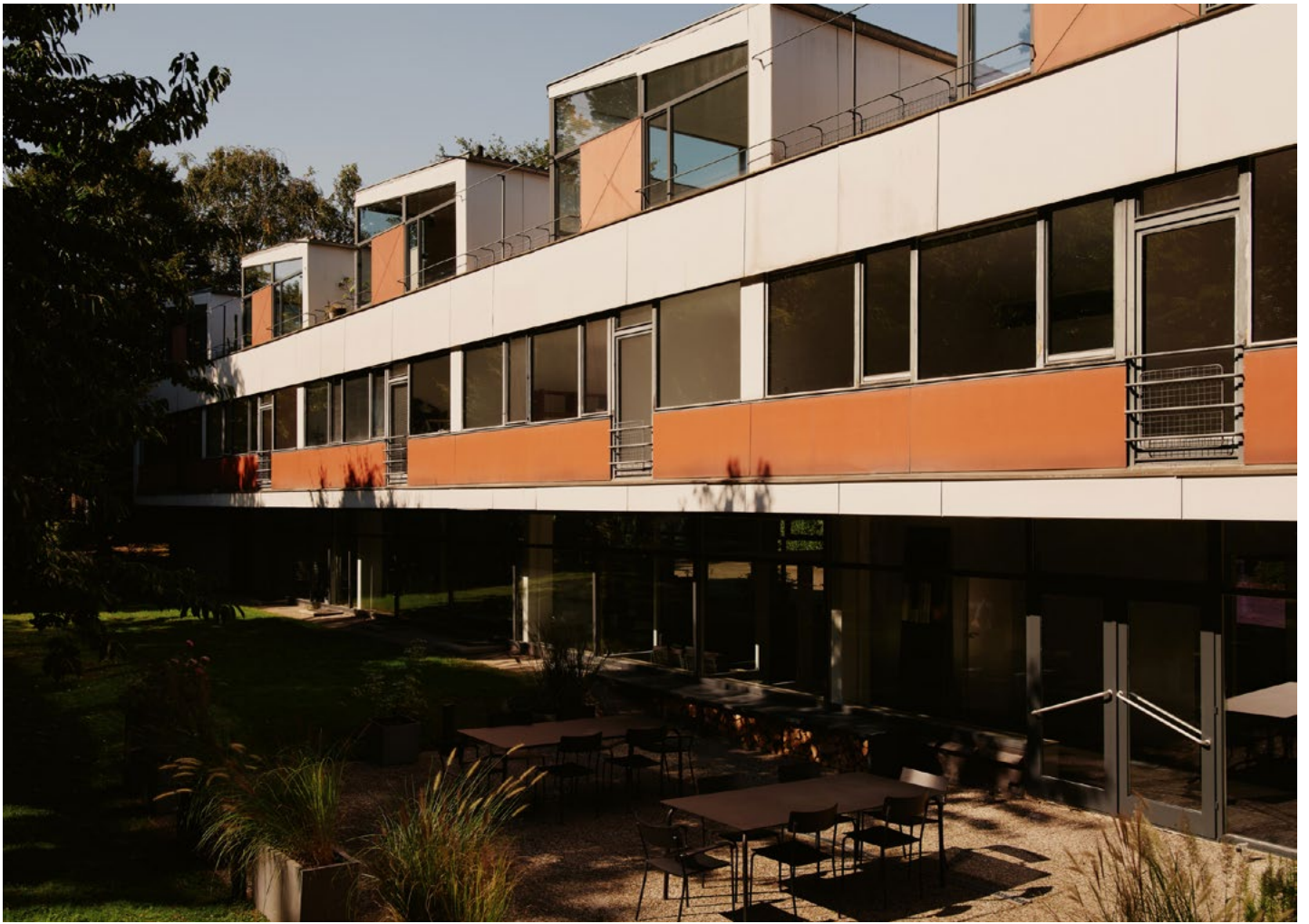
The back of the building has a large terrace in the middle of the Berlin Tiergarten.
