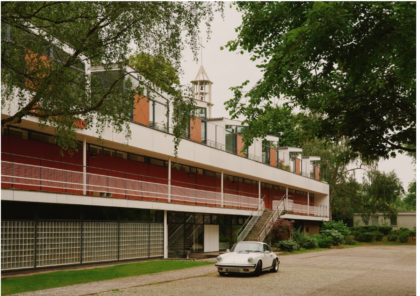
The freestanding Eternithaus has a spacious parking lot for 34 vehicles.
